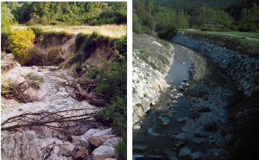
Fig. 9. The Céans river bed in 2004 (left) and in 2011 (right) (Southern French Alps). The bed of the Céans was entrenching strongly in the last decades, due to a great decrease of erosion and sediment transport. The river banks were falling regularly in the entrenched bed (left), obliging the authorities in building new embankments to protect surrounding areas from destruction (right).
